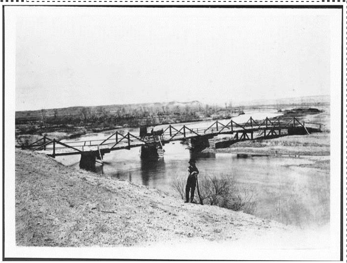
Wagon bridge on the Laramie River in 1868 Photographer unknown University of Wyoming, American Heritage Center
